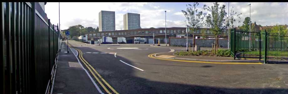
ABOVE: October 2008. The new car park and road layout for Hollingdean Lane
