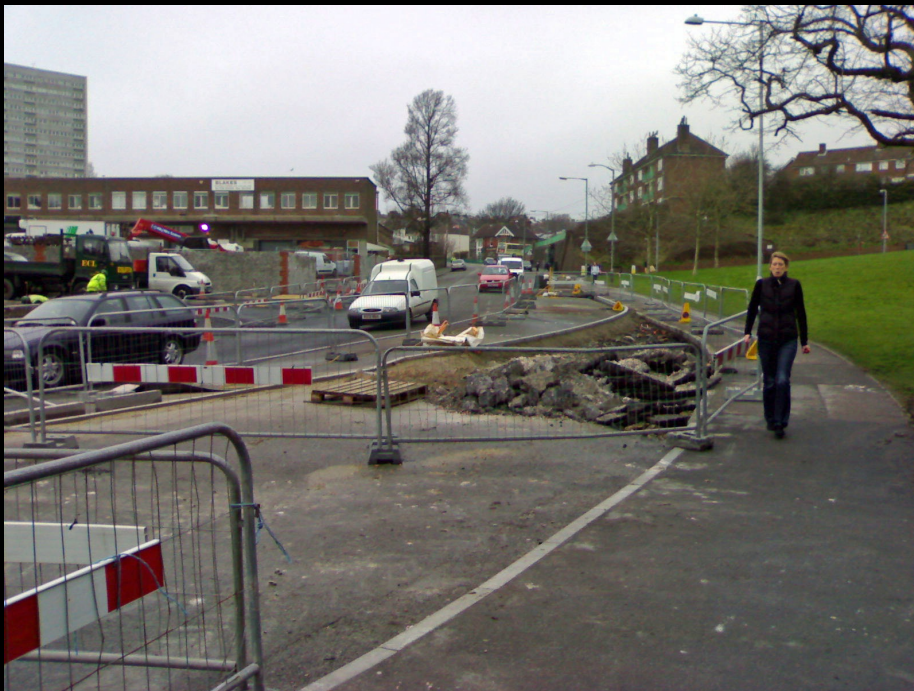
ABOVE: The road at the bottom of Upper Hollingdean Road being widened on 29 th February 2008, to ensure that HGV's do not foul the walls of the tunnel.
