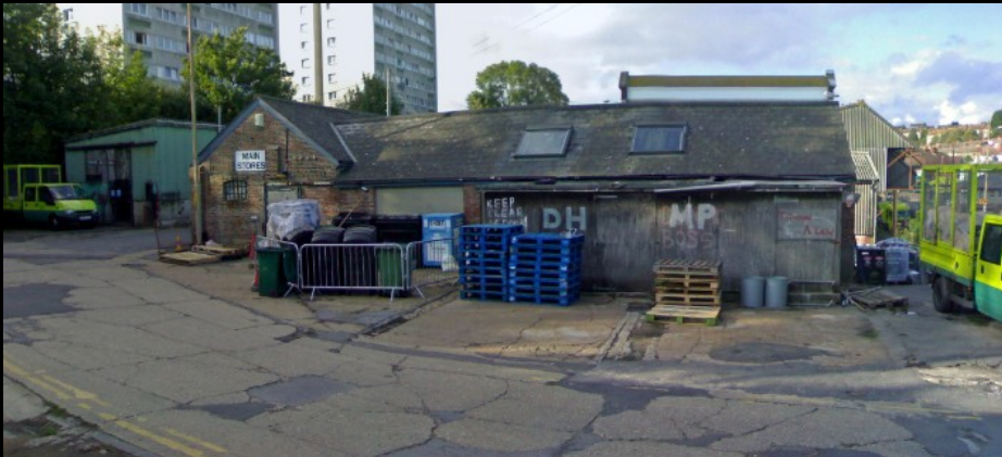
BELOW: This is one of the lesser buildings on the site, but still worthy of note as it has survived unaltered since the time this area was first laid out.
